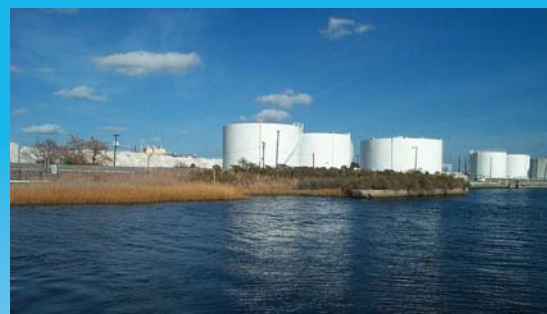
Harbors are vulnerable to flooding and are occupied by industries that use a variety of chemical and petroleum products.
