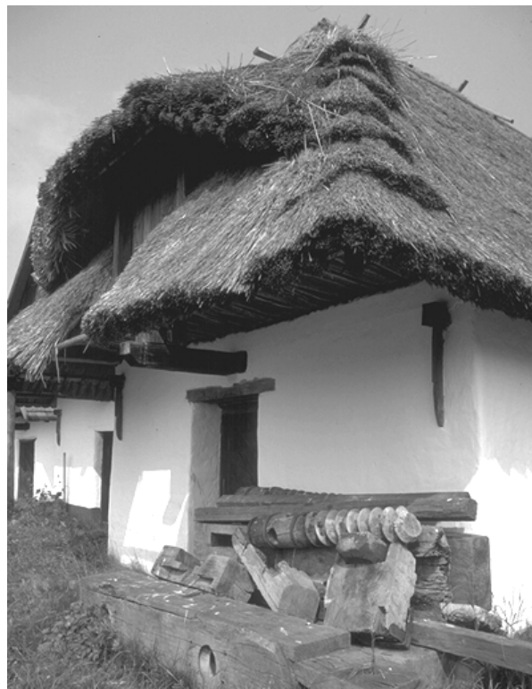
Newly constructed thatched roof.
