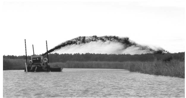
Spray dredging in the Pamunkey River.
