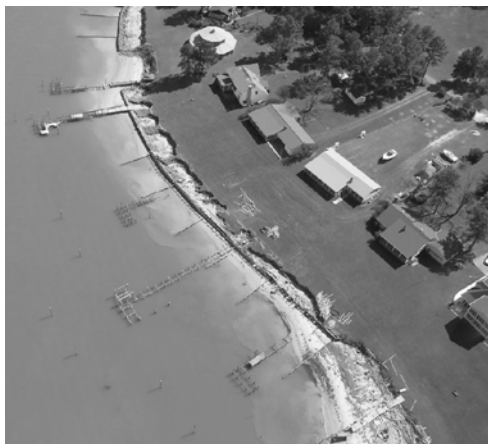
Figure 1. Major erosion and damage to shoreline structures and piers as a result of Hurricane Isabel.
