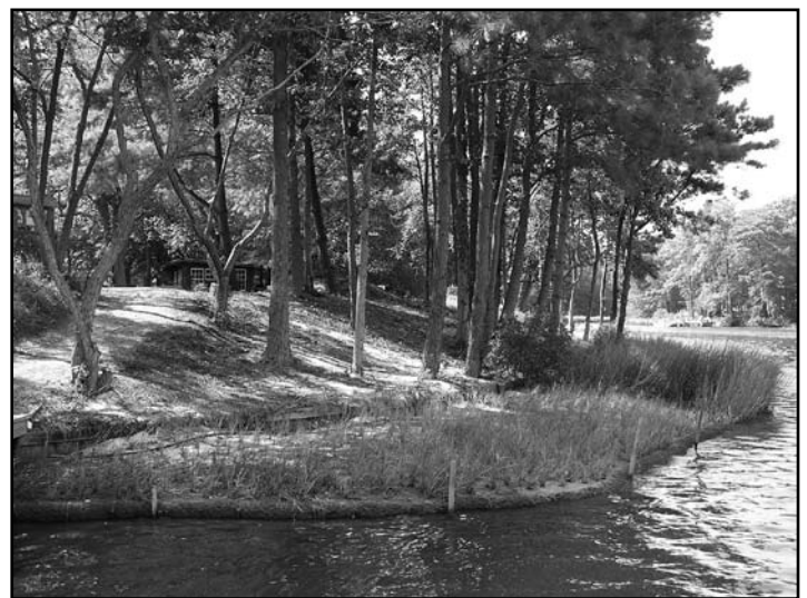
Figure 1. Fiber logs provide temporary soil containment and protection for planted marshes until the root system becomes established.
