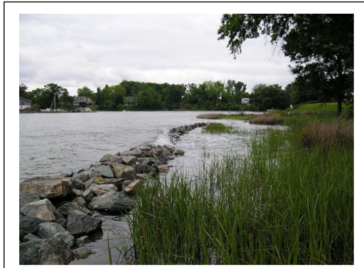
Figure 2. Boat wakes were observed washing over this marsh toe protection structure located in close proximity to a navigation channel. Boat wakes influence the wave climate in low energy settings.
