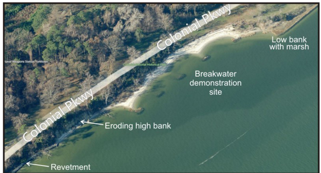
Figure 2-4. Upland bank with revetment, an eroding high bank along the National Park Service's Colonial Parkway.
