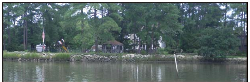
Figure 2-9. Low upland bank in a low-energy residential area that has a rock revetment for shore protection. Photo date 25 Jul 2013.
