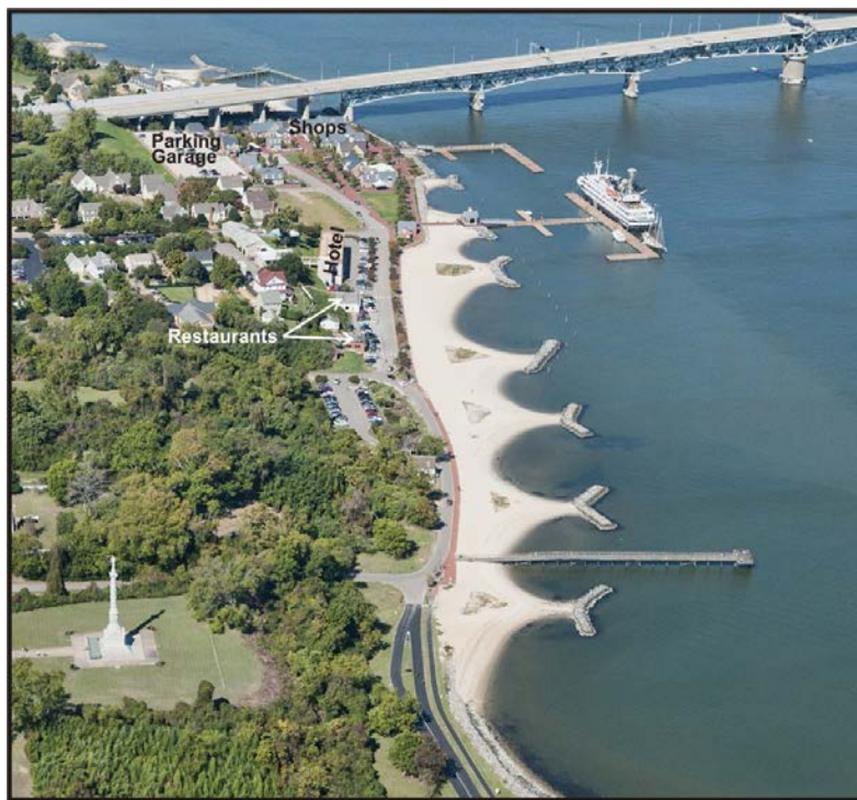
Figure 2-5. Yorktown breakwaters and beach nourishment project. Photo date 17 Oct 2010.
