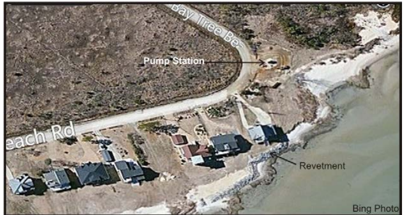
Figure 5-6. Erosion is threatening the sewer pump station for Bay Tree Beach.
