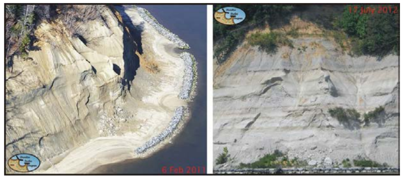
Figure 3-7. High sills built along Westmoreland State Park's high energy, high bank shoreline. The material that slumps from the bank will be caught behind the sills and stabilize the base of the bank by protecting it from wave attack. A more recent photo shows that the slump material is starting to become vegetated.
