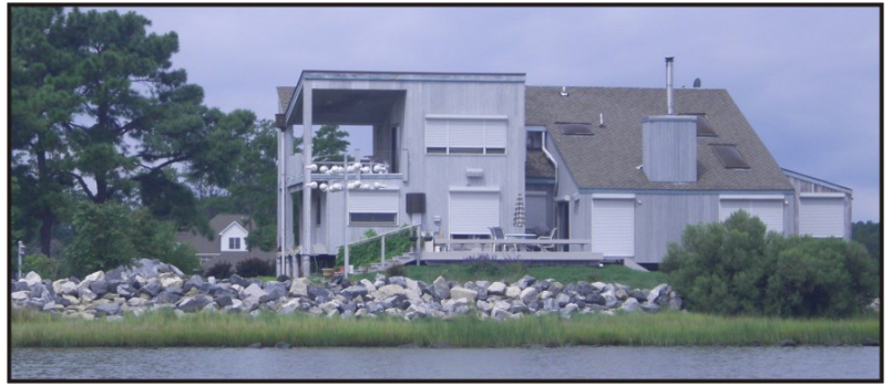
Figure 2-8. Low upland bank in a residential area that has a rock revetment for shore protection behind a fringe marsh
