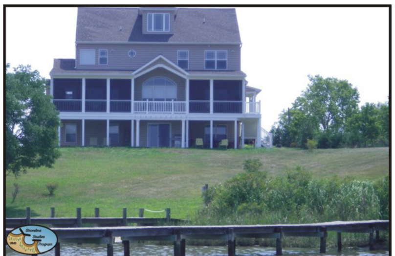
Figure 3-3. Bank grading in Westmoreland County reduces steepness and will improve growing conditions for vegetation stabilization.
