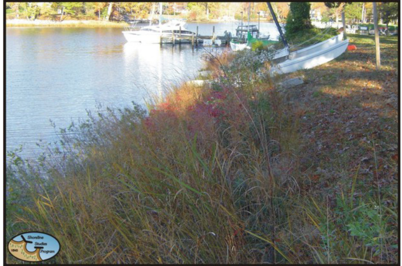
Figure 3-4. This low-energy site had minor bank grading, sand added, and Spartina alterniflora planted. This photo shows the site after 24 years.
