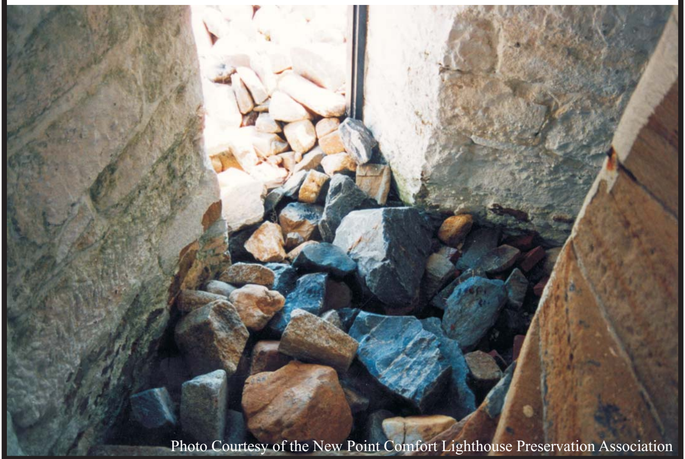
Figure 21. Photo illustrating the present rock revetment's deficiency's and a photo showing how many of the smaller rocks on the island were pushed into the lighthouse during Hurricane Isabel (18 Sep 2003).
