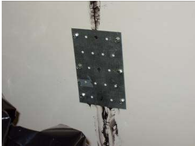
Figure 21: A screw-plate with the appropriate number of screws.
