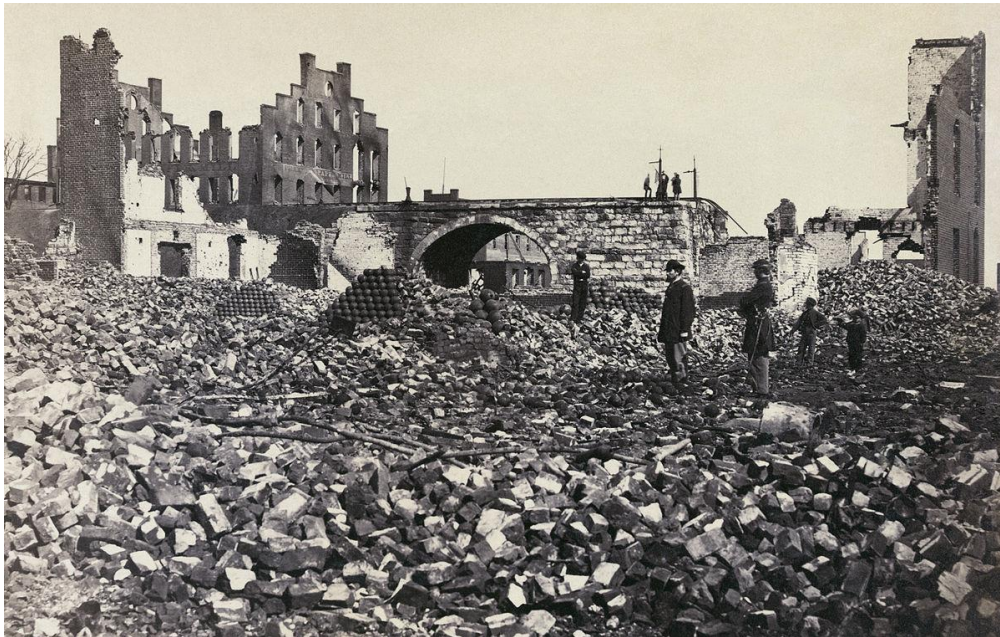
Figure 11 - "Ruins in Richmond" Damage to Richmond, Virginia from the American Civil War by Andrew Russell (1865). (Courtesy of the Library of Congress)
