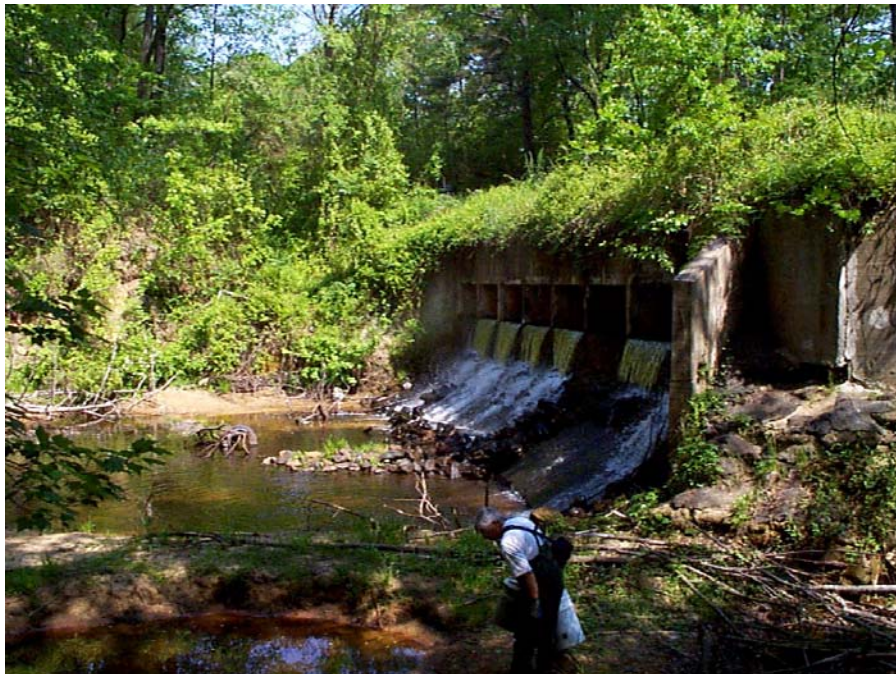
Figure 4. Kamp's Millpond spillway and tailrace. Irish ramp is on far side of creek.
