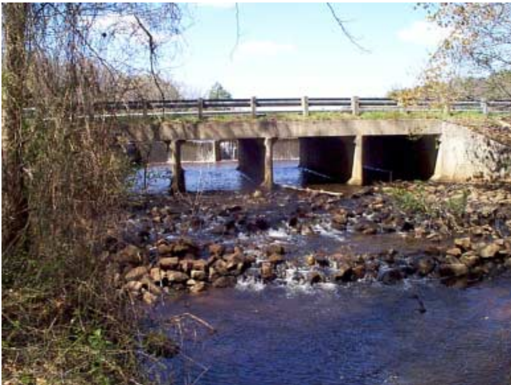
Figure 4. The spillway at Gardy's Millpond (Yeocomico River). The Irish Ramp was located in the culvert on the left.
