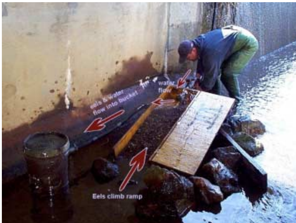
Figure 2. The Irish Ramp at Gardy's Millpond showing its configuration. The arrows indicate the flow of water and eels.
