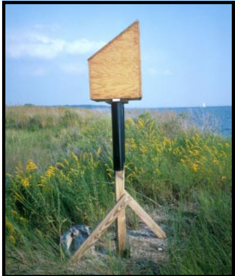
Side view of installed Barn Owl box illustrating posts and sheet metal predator guards. Note the toe and diagonal side braces. Photo by David Whalen.
