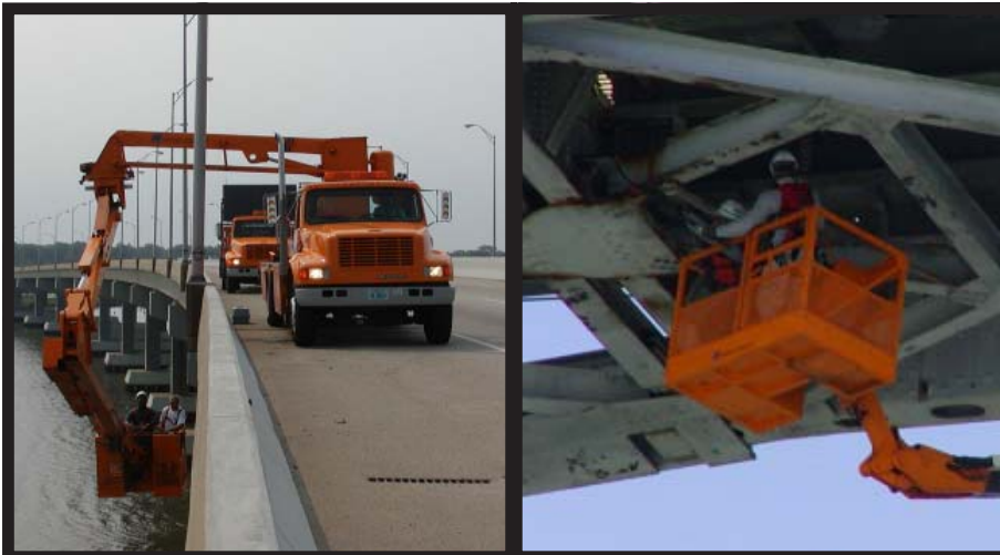
Access to some bridge nesting sites is not possible without specialized equipment. Boom truck used to access West Norfolk Bridge (lft) and Norris Bridge (rt). Photos by Bryan Watts and Bart Paxton.
