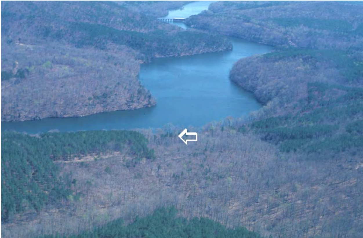
Figure 12. Overview of Nest ST-01-02 with Falls Dam in the background.
