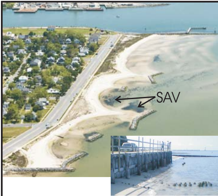
A breakwater system is effective shore stabilization on higher energy shorelines. The system can create or enhance a living shoreline with beach fill and dunes. Submerged aquatic vegetation (SAV) has taken root in the embayments and in the lee of the structures. Inset: The exposed bulkhead was hazardous before stabilization with a living shoreline strategy. Cape Charles, Northampton County, Virginia, May 2009 (Inset August 1999)
