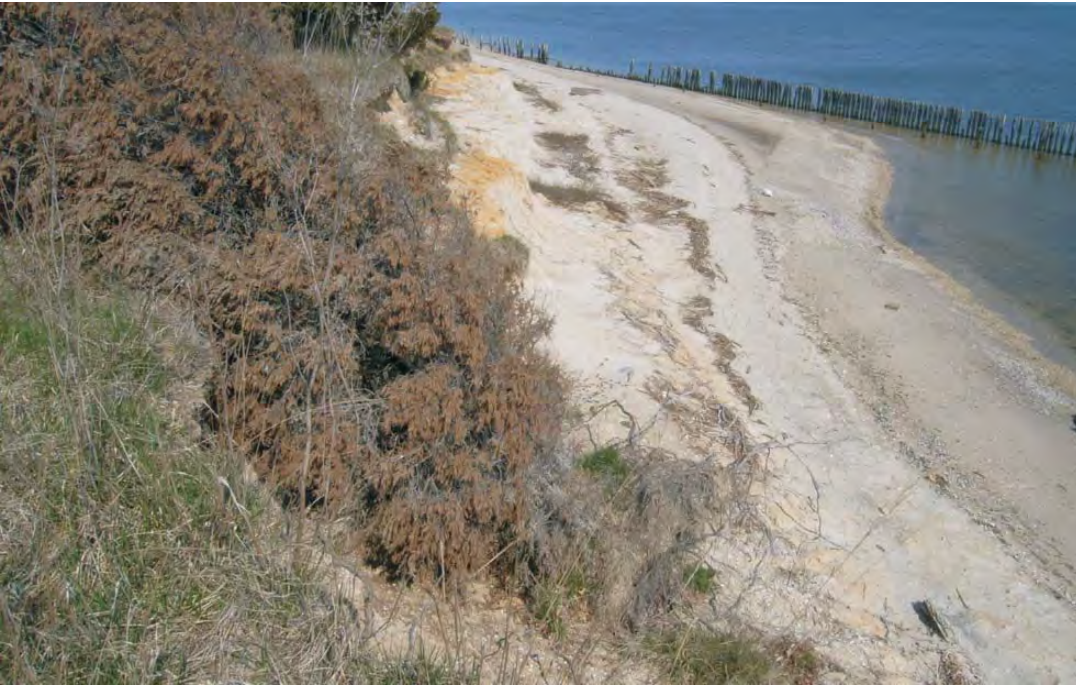
19. Along the northeast facing shoreline north of the sandy spit - Remnants of an old bulkhead are
