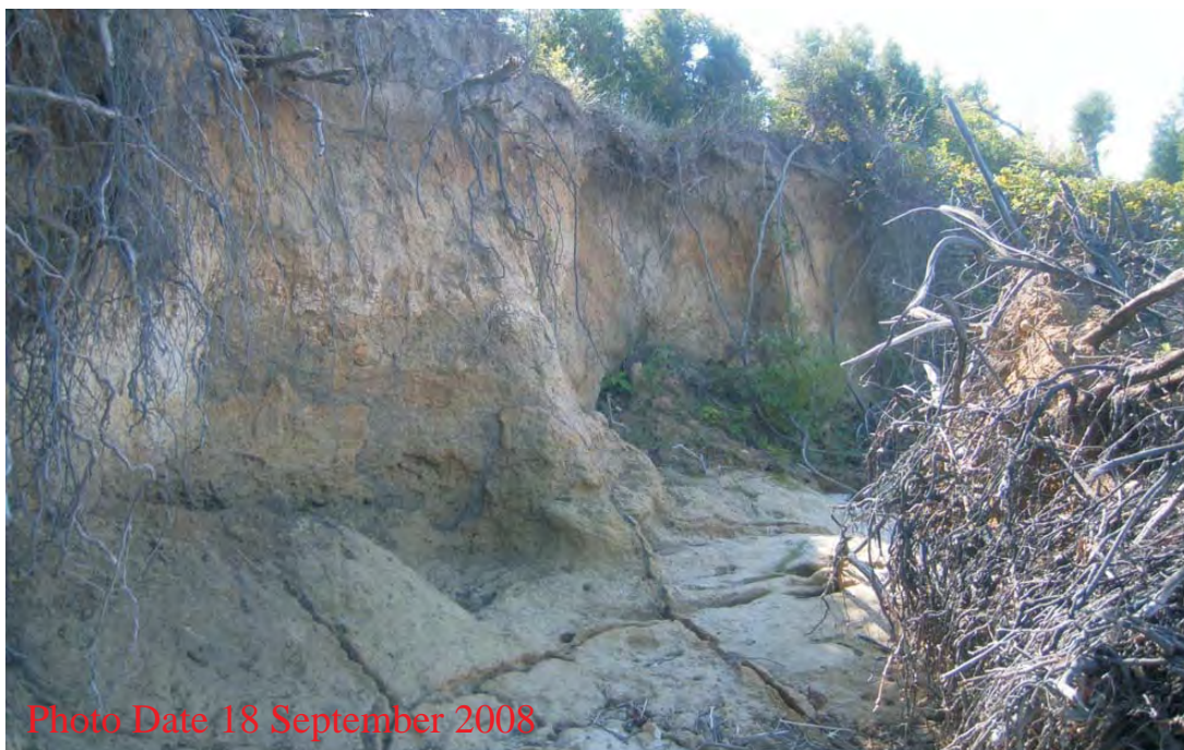
9. Erosional headland west of Digwood Swamp
