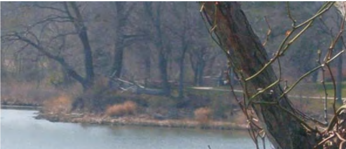
30. Eroding point of land near the Visitor's Center.
