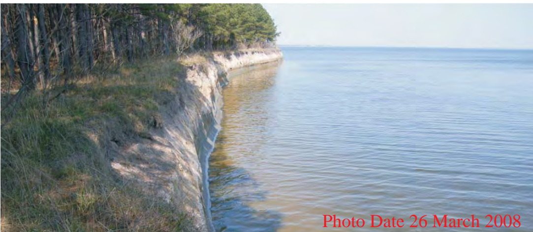
15. Vertical banks with no beach at high water along forested embayment - Top of bank elevation varies due to erosion at the top
