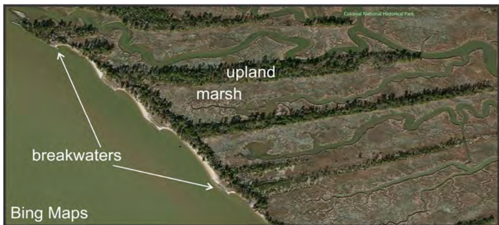
Figure 3-8. Bing map showing headland breakwaters that were built along Jamestown Island's James River shore.
