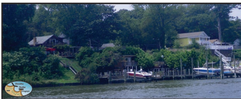
Figure 2-11. The shorelines along this section of shoreline in Reach 2 along the Potomac River has been graded and protected at the base.
