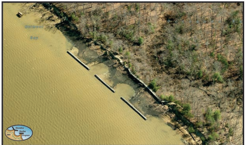
Figure 2-8. Gabion structures that are acting as breakwaters along Mason Neck State Park. From Bing Maps.
