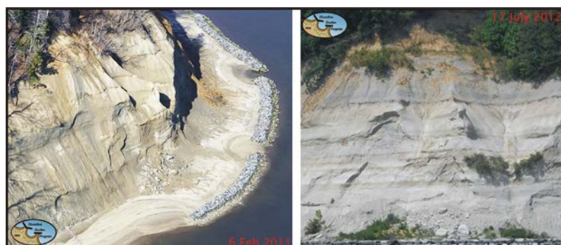
Figure 3-7. High sills built along the Potomac’s high energy, high bank shoreline. The material that slumps from the bank will be caught behind the sills and stabilize the base of the bank by protecting it from wave attack. A more recent photo shows that the slump material is starting to become vegetated.
