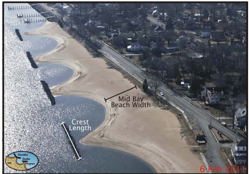
Figure 3-8. The breakwaters at Colonial Beach provide a wide recreational beach as well as storm erosion protection for the residential upland. These structures were installed in 1982.
