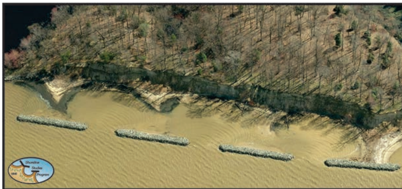
Figure 2-9. One attached and three detached breakwaters along Mason Neck north of High Point. As the sandy bank erodes, the breakwaters likely will become attached. From Bing Maps.
