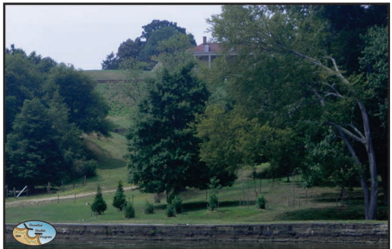
Figure 2-15. The high bank at Mount Vernon has been graded and the shoreline protected with a stone block seawall.
