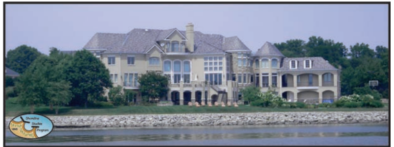
Figure 2-14. Ferry Point differs from other points in Fairfax in that it is developed and protected with a large revetment.
