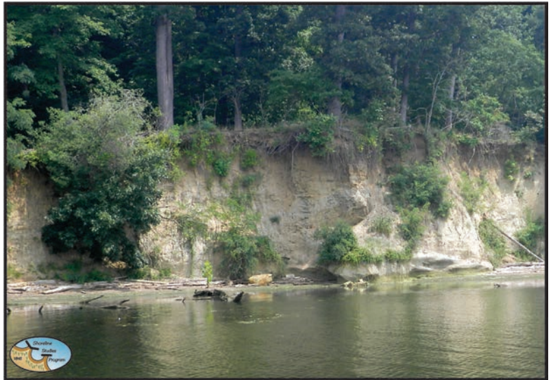
Figure 2-7. Eroding banks along Belmont Bay.
