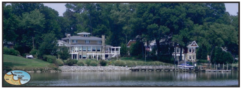
Figure 2-13. Development and shore protection along Dogue Creek.
