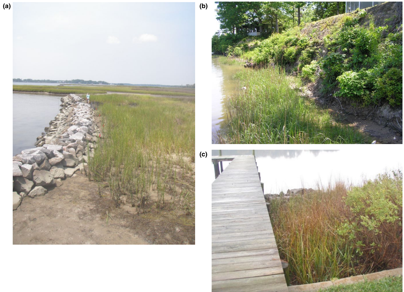
FIGURE 2 Comparison of retreat potential for living shorelines. (a) This living shoreline was constructed adjacent to natural marshes and on a low elevation shoreline with ample opportunity for retreat. However, the somewhat sparse grass may limit its ability to accrete sediment. (b) This marsh is in front of a bluff, which cuts off the retreat pathway but provides sediment for accretion. (c) This living shoreline is built in front of a block retaining wall that cuts off the retreat pathway. Survival under sea level rise will require sufficient sediment accretion to maintain its elevation within the tidal frame
