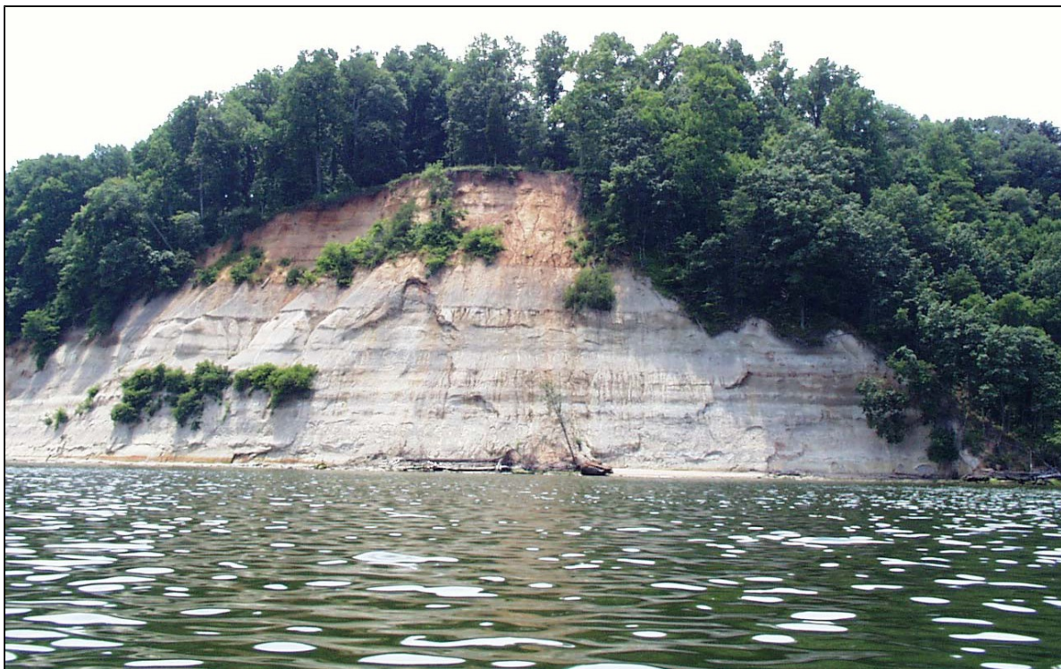
Figure 6. Horsehead Cliffs in Westmoreland County, Virginia
