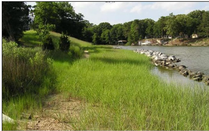
Figure 3. Living shoreline example includes a well graded vegetated bank, a planted marsh with a marsh sill to protect the toe of the marsh.
