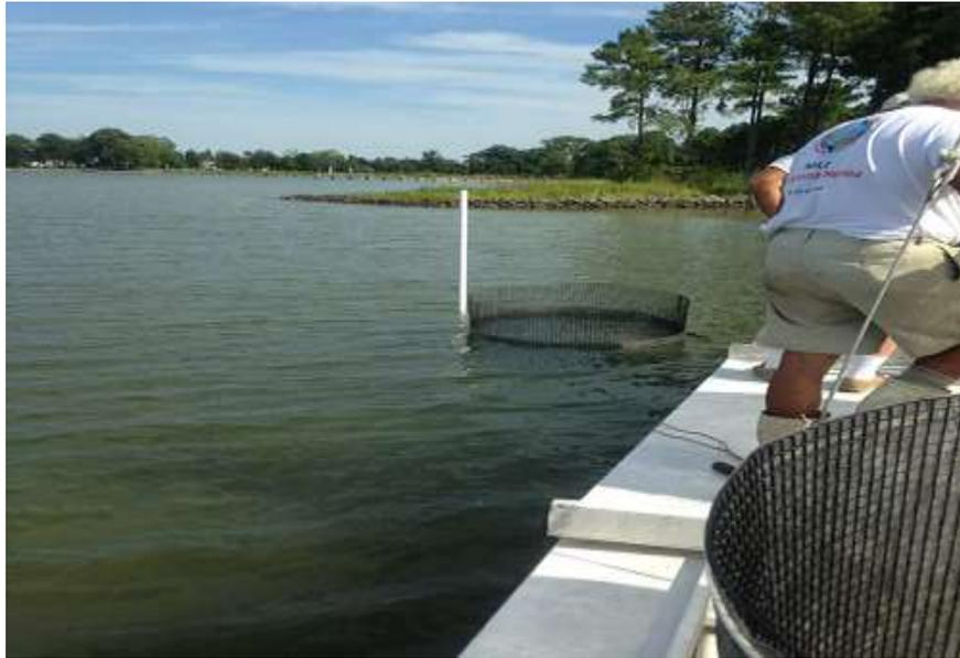
Photo #1: Wire cylinders being installed in Cranes Creek on 08/21/13. Note the filter cloth, just visible above the water. Photo courtesy of Karen Hudson.
