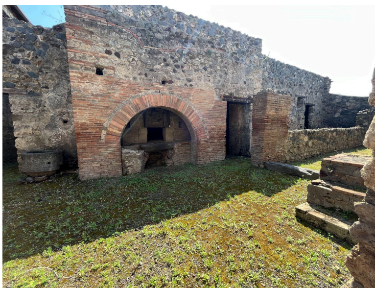
Fig. 22. Oven room (E) of mill-bakery I.12.1-2. Photo by author.
