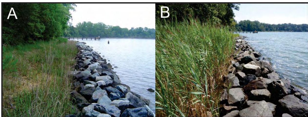
Figure 4-3-7. Sill at St. Mary's A) five years after construction (9 May 2007), B) 16 years after construction (15 Aug 2018). Phragmites has colonized behind the structures.
