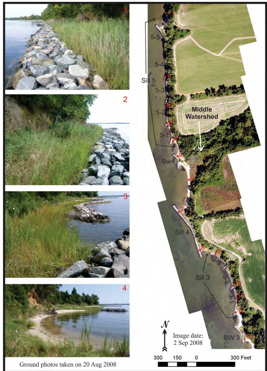
Figure 4-4-2. A photo mosaic of Jefferson Patterson Park & Museum shoreline on August 20, 2008 depicting the location of sills and breakwaters and indicating the locations of the ground photographs.
