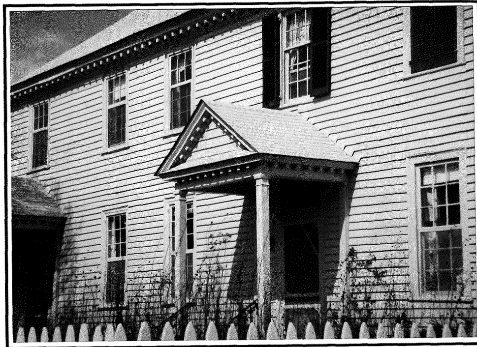
Figure 19. Timberneck, Structure 36-74, detail of front porch with pedimented and modillioned roof.
