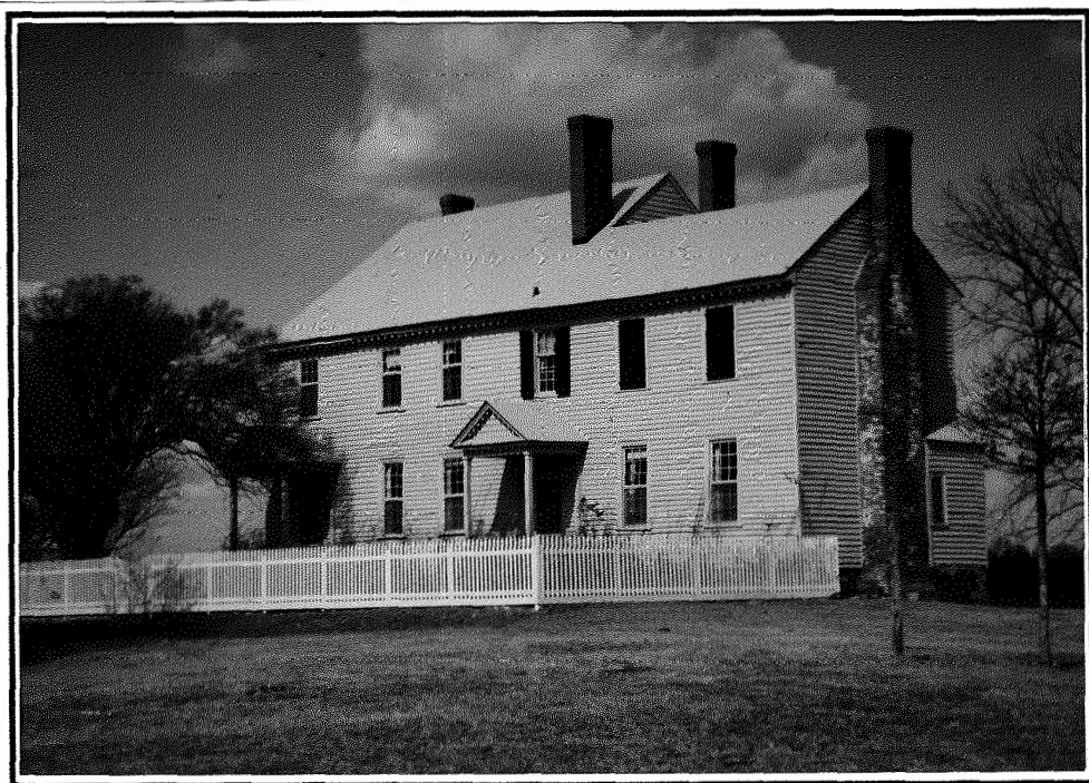
Figure 18. Timberneck, Structure 36-74, north and east elevations.
