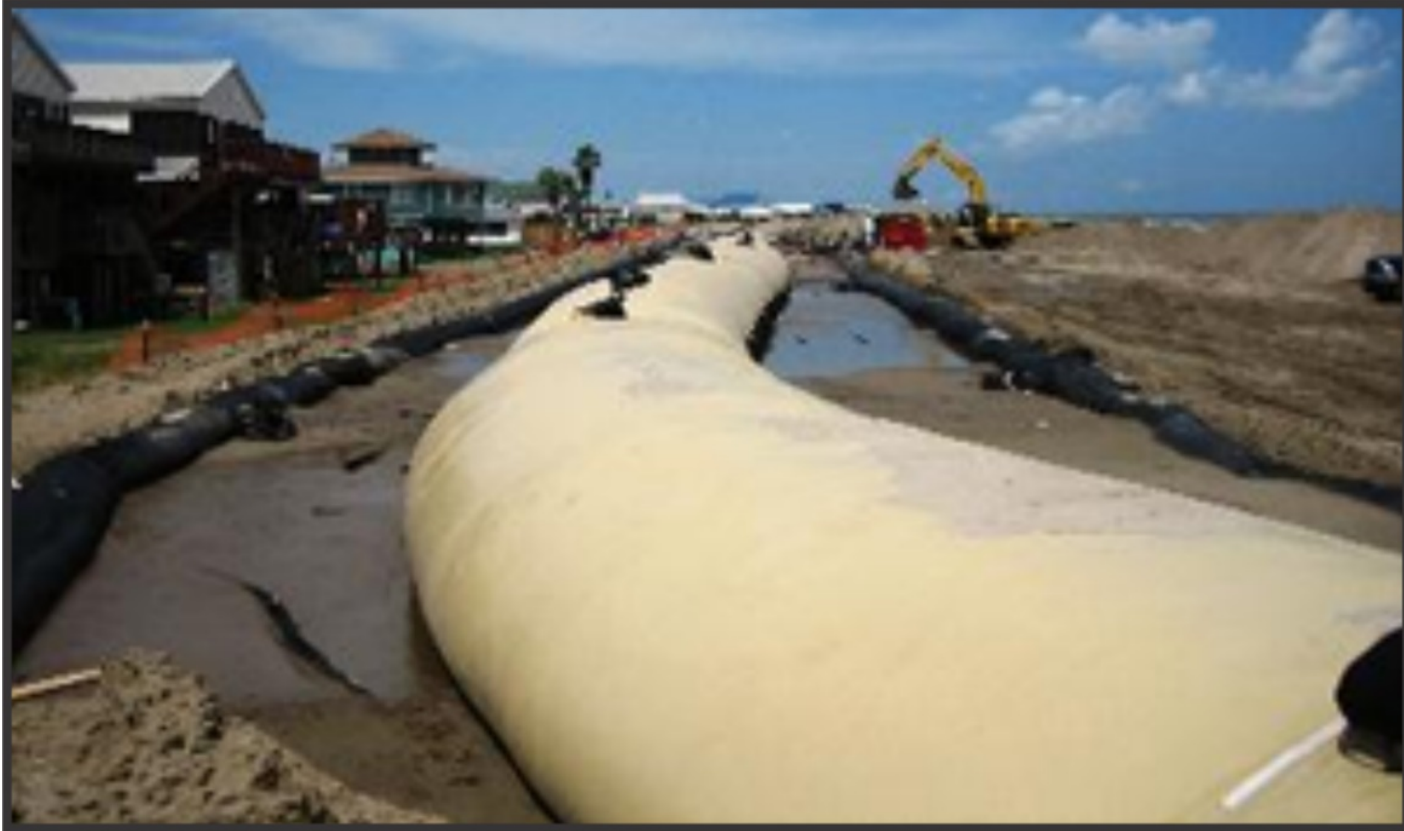
Figure 14. Example photo of a Geotube used for sediment containment. Source: TenCate website
