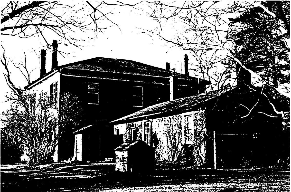
Figure 5. Benares, Back View showing 1835 Kitchen Ontario Heritage Foundation
