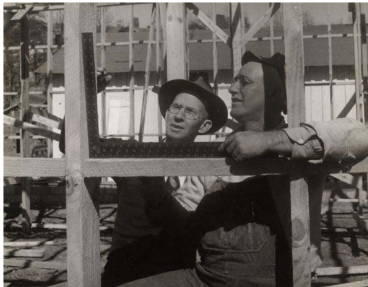
Figure 29, From WHS, "Two men working on the construction of a building at Highlander Folk School." Wisconsin Historical Society, "Building at Highlander," 52399. Viewed online at https://www.wisconsinhistory.org/Records/Image/IM52399 .
