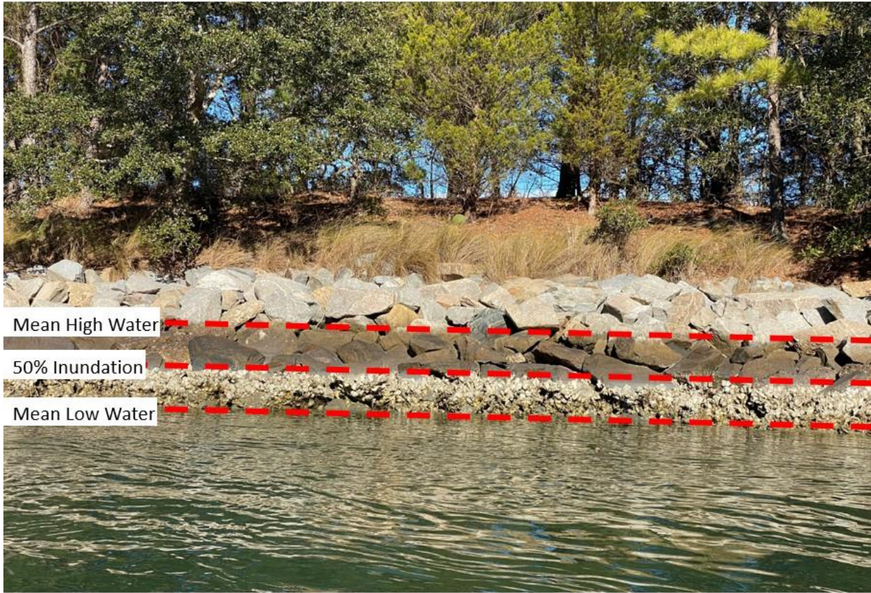
Figure 15: Showing the threshold of oysters growing range between MLW and MHW. This image was taken on the Lynnhaven River. K. Grigsby, 2023.
