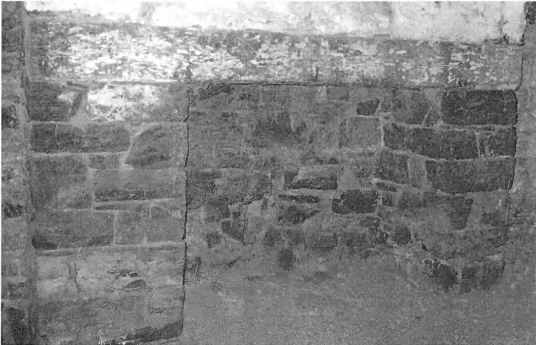
Figure 21: Redwell office, Wood lintel, First Floor Fireplace
