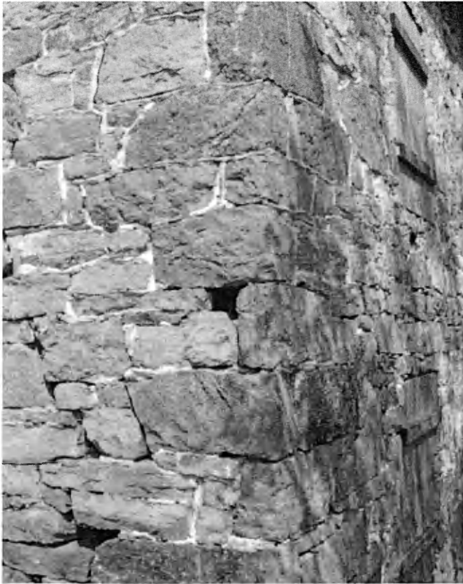
Figure 19: Redwell office, Prism Mortar Joints
