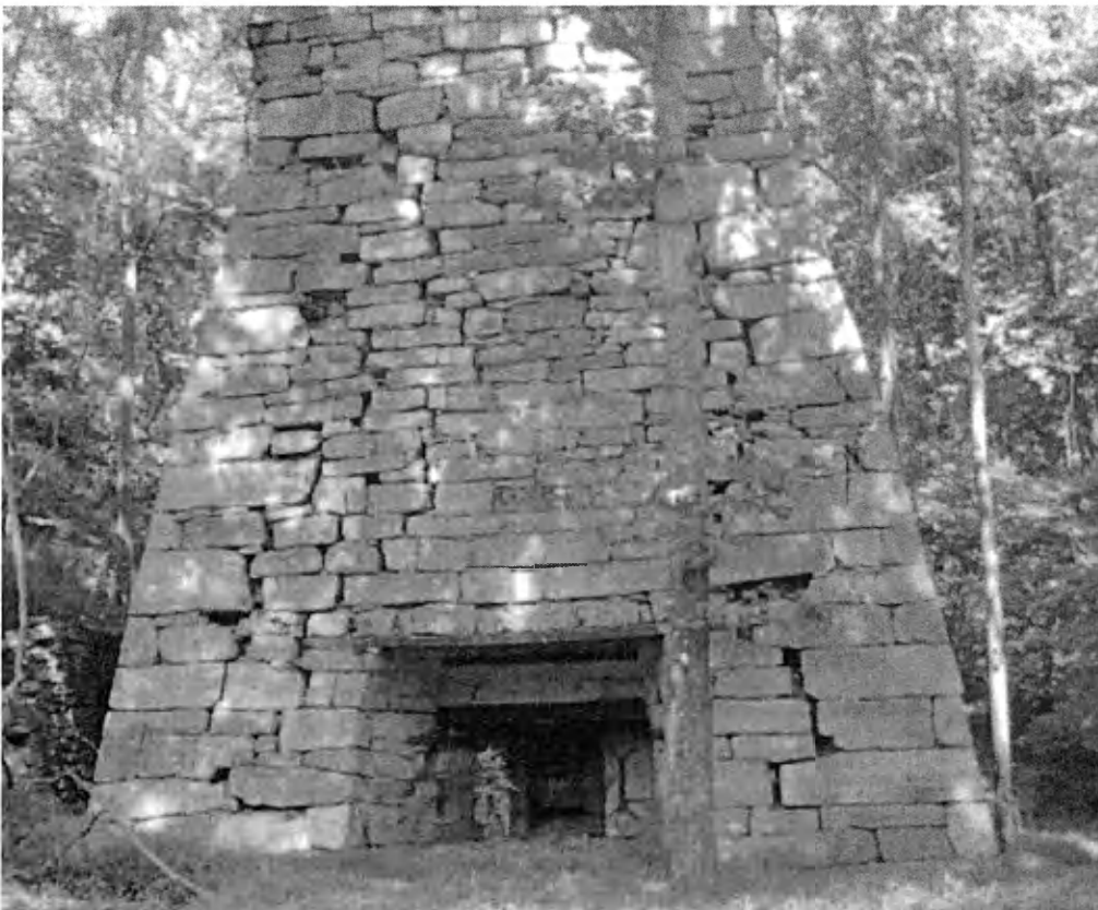
Figure 24: Van Buren Furnace Stack, Shenandoah County, Virginia
