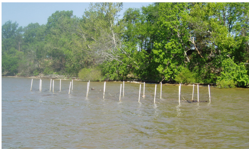
Figure 7. SAV restoration enclosure on the Upper James River. Enclosure fencing consists of 1.5-in. PVC poles and 1-in. mesh polyethylene aquaculture netting.
