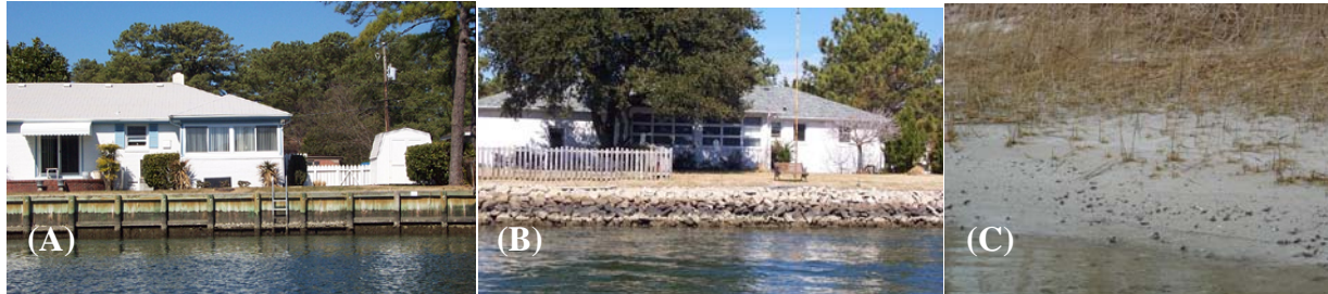
Figure 31. Examples of (A) bulkhead, (B) riprap and (C) sand habitat.
