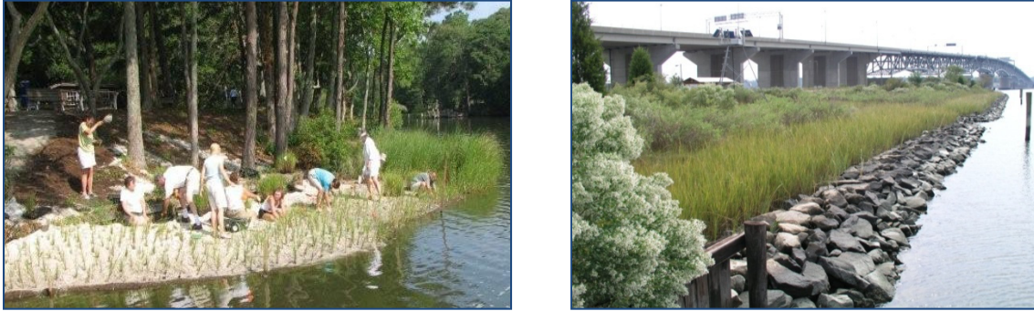
Figure 1. Non-structural living shoreline marsh planting (left) and hybrid living shoreline with planted marsh and rock sill (right).
