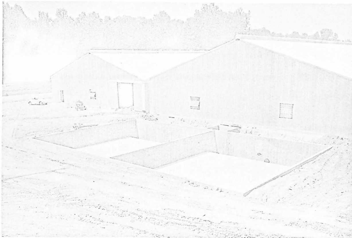
Fig. 2. Showing building housing the James River hydraulic model and the water supply facility. (Courtesy of U.S. Waterways Experiment Station, Vicksburg, Mississippi.)
