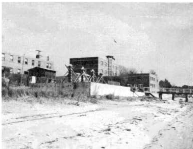
4 - MICROBIOLOGY LABORATORY (Under construction Feb. 1961)
