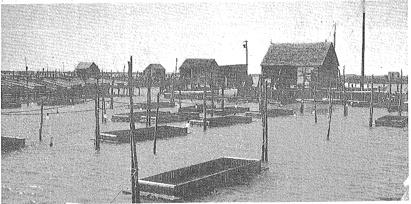
The center of the float operation is a wooden building supported on pilings and surrounded by floats tied to stakes in the water.
