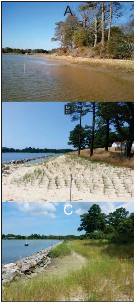
Figure 4-2-6. Photos of reach 3 at Occohannock on the Bay A), before construction (March 2013), B) after planting (May 2013), C) after 5 years.
