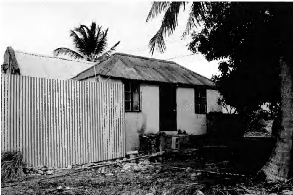
Plate 3: Another stone house located in St. Lucy, constructed of cut, coral limestone blocks. The technique of sawing coral stone into blocks was a post emancipation development.
