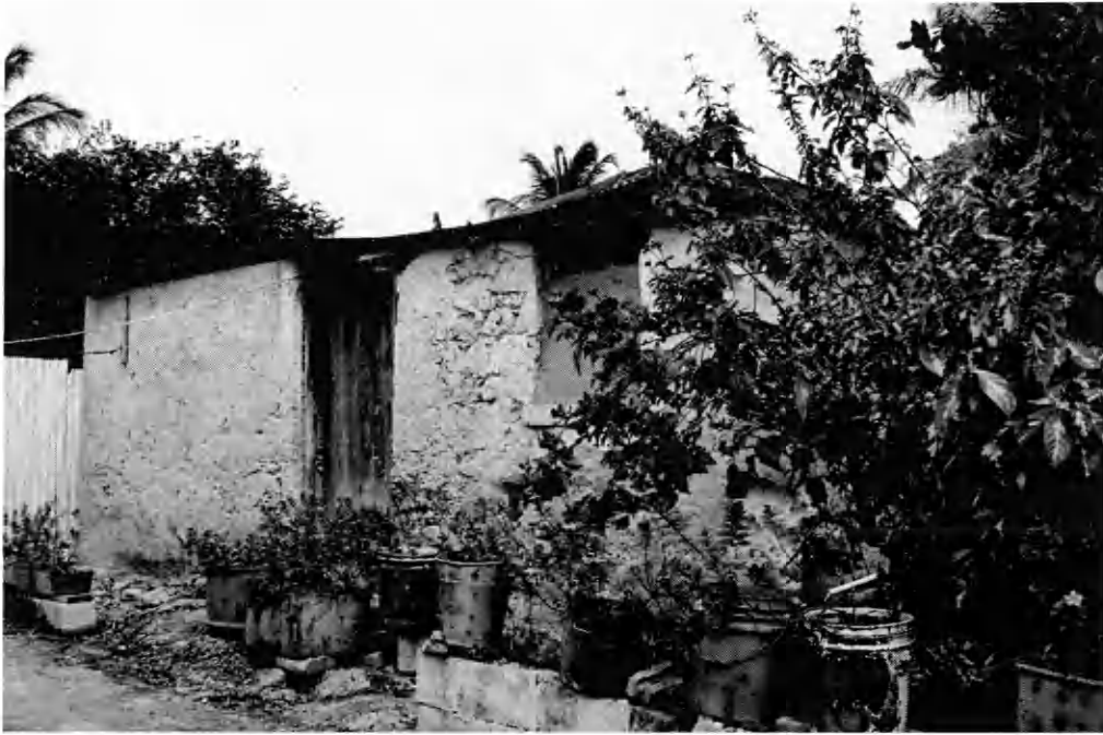
Plate 2: One of a handful of rubble stone houses located in the parish of St. Lucy, all showing diversity in architectural features from the Moore Hill house. This house is built on a stone foundation to provide a water table.
