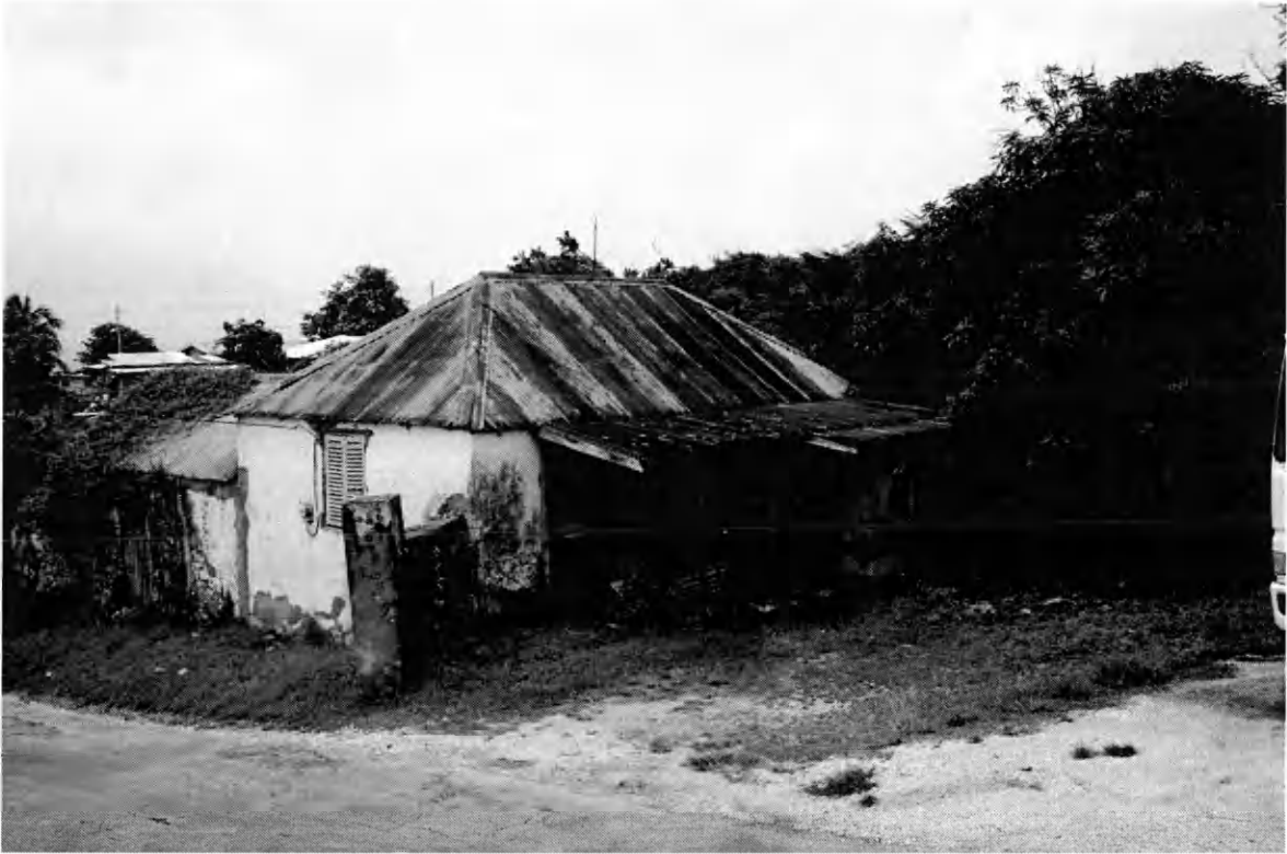
Plate 6: A rubble stone house in the rural, northern parish of St. Lucy. This house has many later additions built on, but it appears the oldest part of the structure was in the rear. This house is not located in a plantation tenantry, suggesting it was constructed in the nineteenth century by small land holders.
