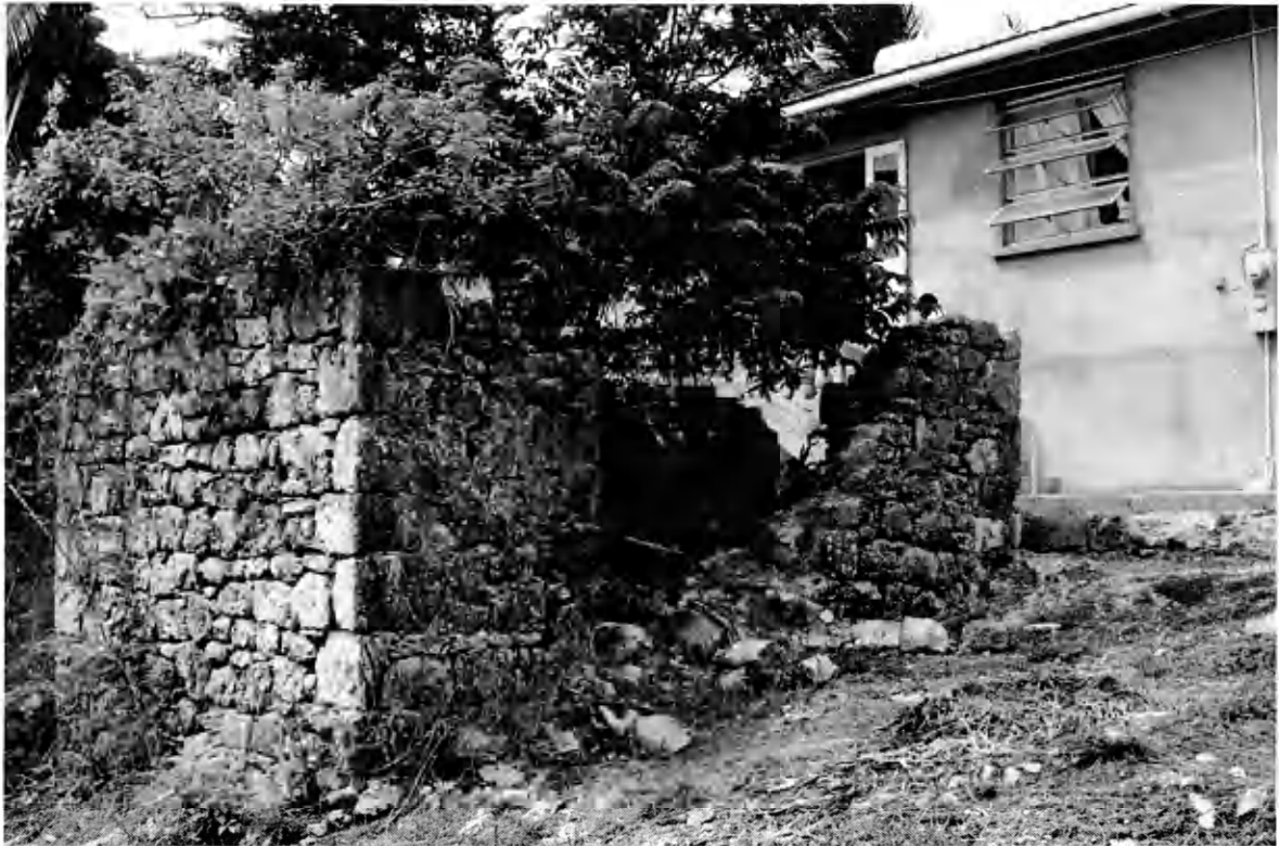
Plate 4: A very small rubble structure without limestone mortar, located in St. Lucy. This structure was likely used as a kitchen, and would have been located behind the house.
