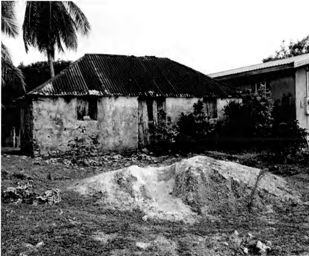
Plate 1: The Moore Hill house, constructed of rubble coral limestone, is located on the western periphery of St. Nicholas Abbey estate.
