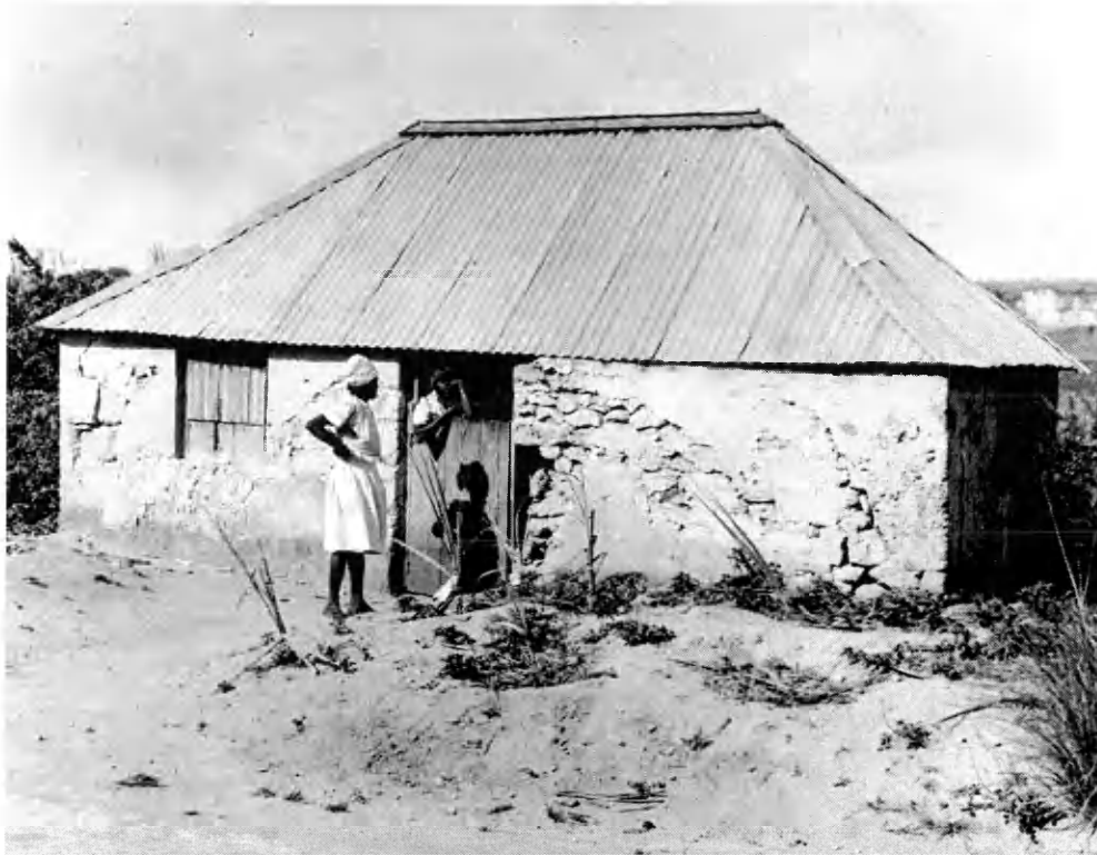
Figure 7: Stone house of rubble construction, with limestone exterior plaster and galvanized hip roof. Photo was perhaps taken in the 1940s or 1950s, but location is unknown (Handler and Bergman 2009: 8).
