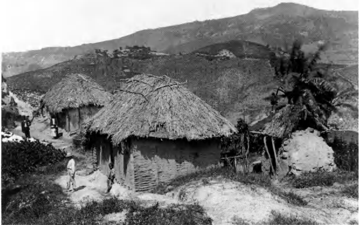
Figure 8: Wattle and daub houses with thatched roofs, probably very similar to those found during slavery. These houses appear to be located in the rugged Scotland District located in the parish of St. Andrew, and possibly the village of Chalky Mount (a pottery kiln is in the lower right hand corner). The American photographer Frank Carpenter (d. 1924) took this photo (Handler and Bergman 2009: 6).
