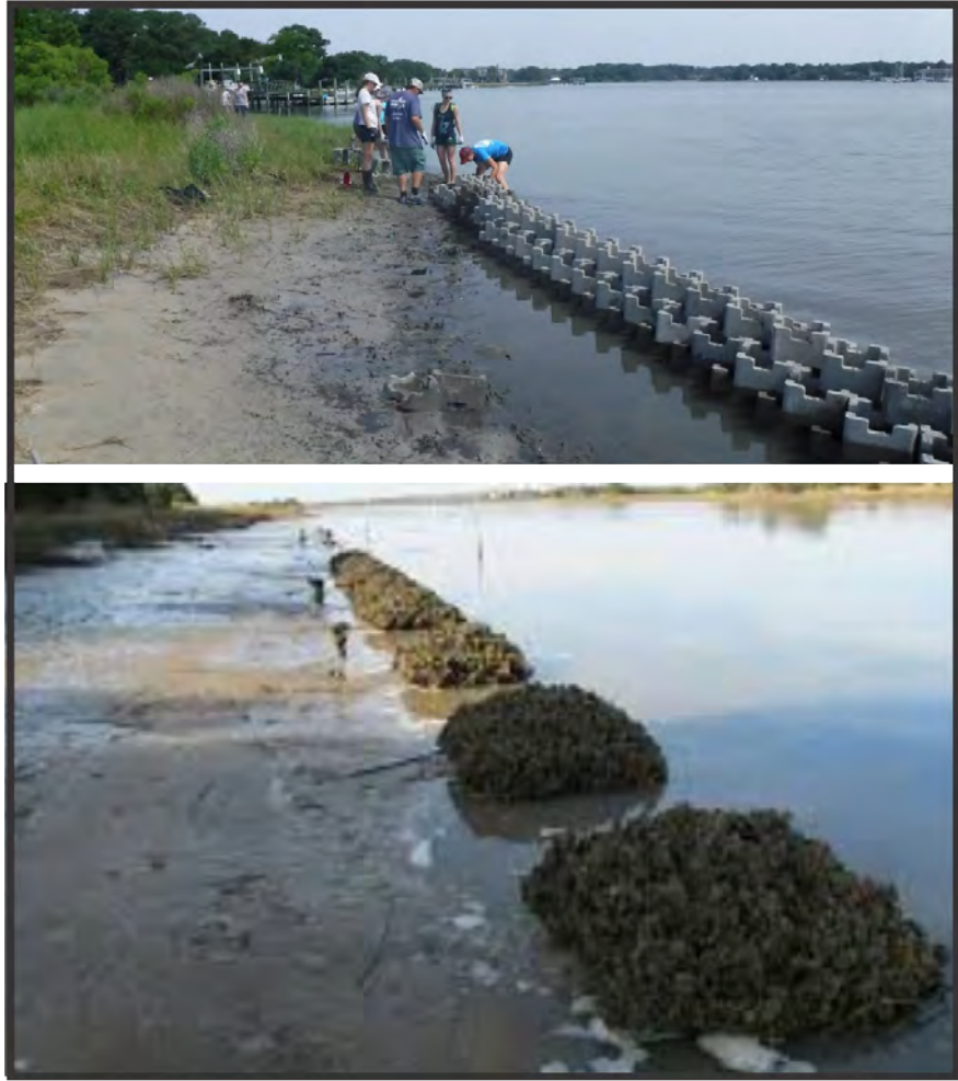
Figure 8. Example of oyster castle placement in an estuarine environment (Photo from Allied Concrete). The top image shows what the reefs look like when first placed. The bottom shows the reefs after oyster recruitment. The proposed structures for Hog Island are higher and wider than this oyster castle sill.
