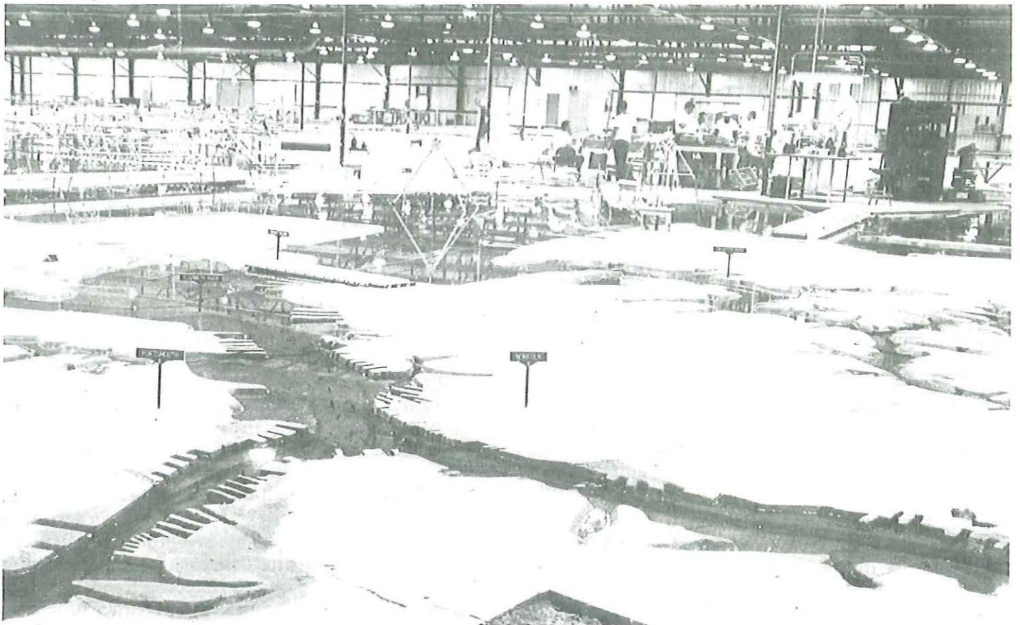
Various stages of model construction: templates were lowered into ground and concrete molded over them. Hydraulic resistance strips protrude from model bed (upper left). VIMS scientists conducted field studies of the James River to gather hydrographic information needed for model construction and verification (upper right). View inside shed where model is housed: salinity withdrawal apparatus appears in left background, tide gauge in middle background, and tide control mechanism (clocklike) in right background.
