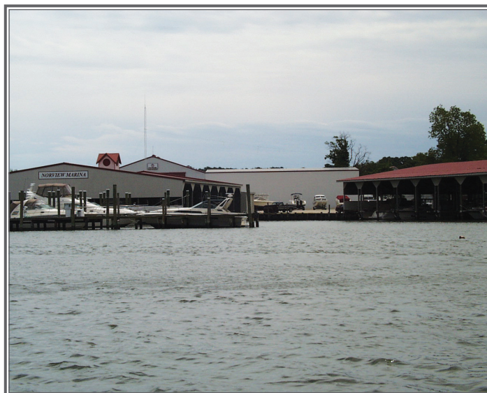
The complex infrastructure associated with marinas places them in the category "Area of Concern" where they require special consideration.
