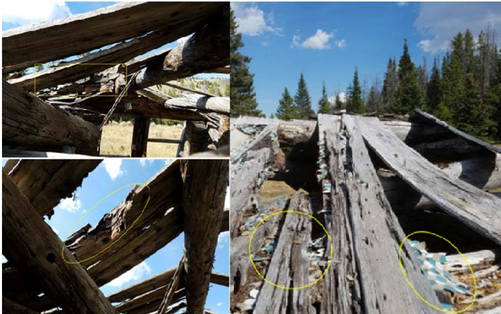
Figure 7.17: Insulation Attached to Roofing Beams, Found During Pedestrian Survey at Highland City
